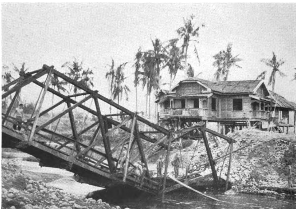
Top: The muddy roads inside Ormoc present almost as troublesome an obstacle as the Jap. Bottom: One of the many bridges knocked out by the U. S. Army Air Forces. Another job for the Engineers!
