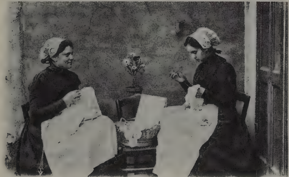
Embroiderers working at home. Women workers tended to be concentrated in a few sectors of the wage-earning economy, especially those involved in the production of textiles and clothing. Much of this work was done at home, where it could be accomplished along with domestic tasks. Bibliothèque Forney, Paris.
