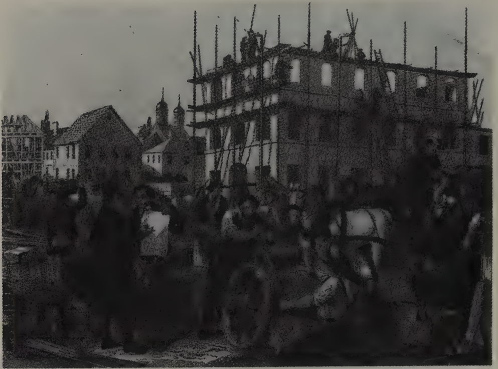
Construction site. Workers unload materials, mix and carry mortar, and, in the distance, erect the building, while the contractor and owner consult in the foreground. Bibliothèque Forney, Paris.
