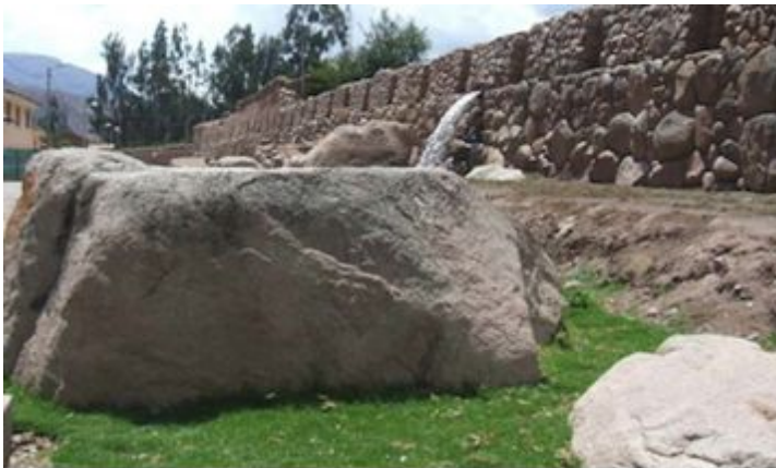
Figure 15: The massive southern wall of Quespiwanka with 40 double jamb niches and a shaped granite boulder in the foreground (photo by the author).
